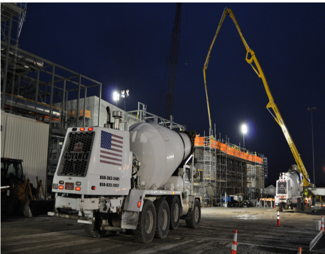
The munitions demilitarization building's final concrete placement was performed on the unpack area.
