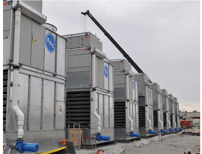
Water will be cooled by evaporative coolers to support plant processes.
