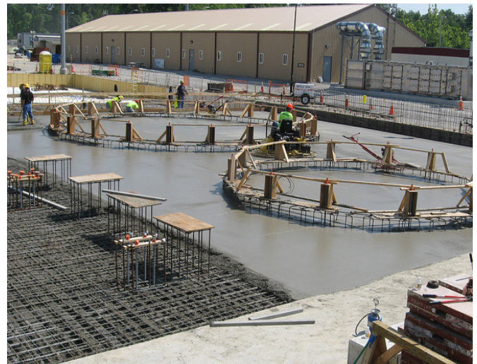
Recent concrete work has involved the hydrolysate storage area.
