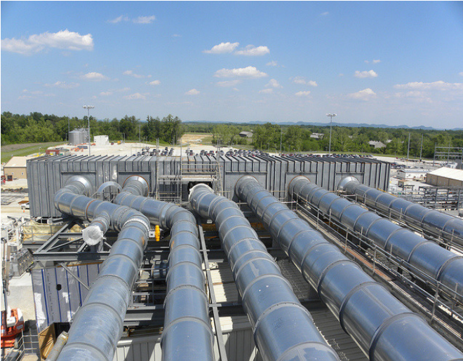
The cascading ventilation system ducts stretch across the control and support building.
